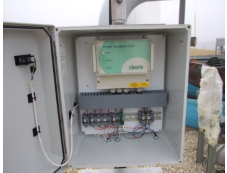
Field Mounted SureSense Controller at Rio Vista
