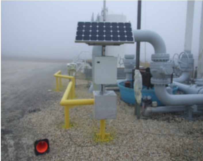
Solar Panel Field Installation at Rio Vista
