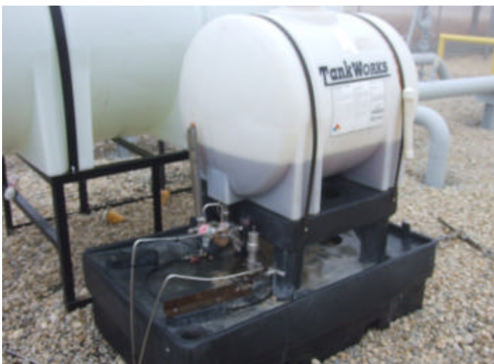
Anti Foam Dosing Skid & Pump at Rio Vista
